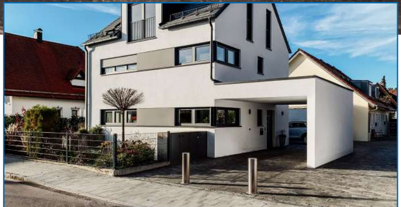
Installation in Munich, Germany Installation in München, Deutschland
