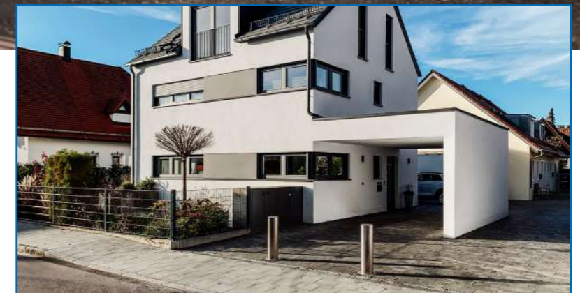
Installation in Munich, Germany Installation à Munich, Allemagne
